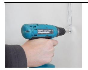
Stretched chain has to be fixed to the wall by adjusting the added safety element – on the height 150cm from the floor minimum. If necessary adjust the chain length.
